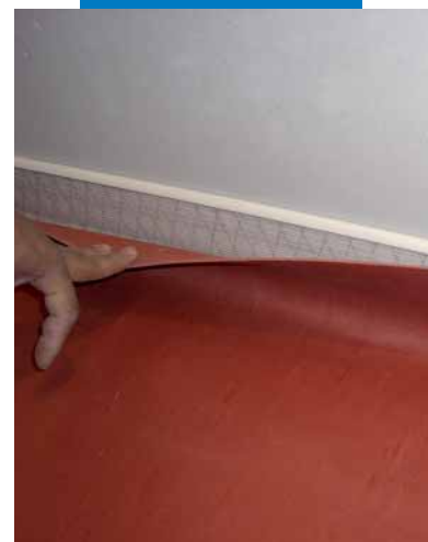
Forming a fillet shell using Mapecoat
